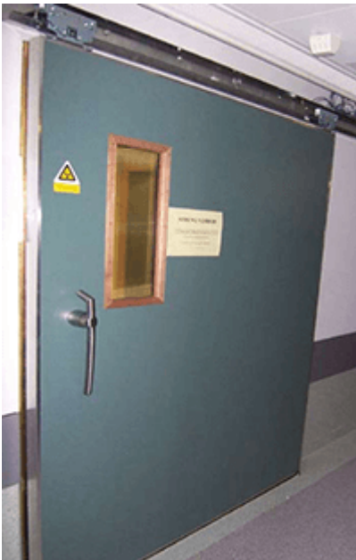
Shielding Faraday cage sliding door
