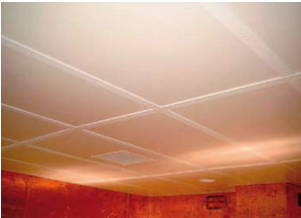
Mu-copper detachable ceiling
